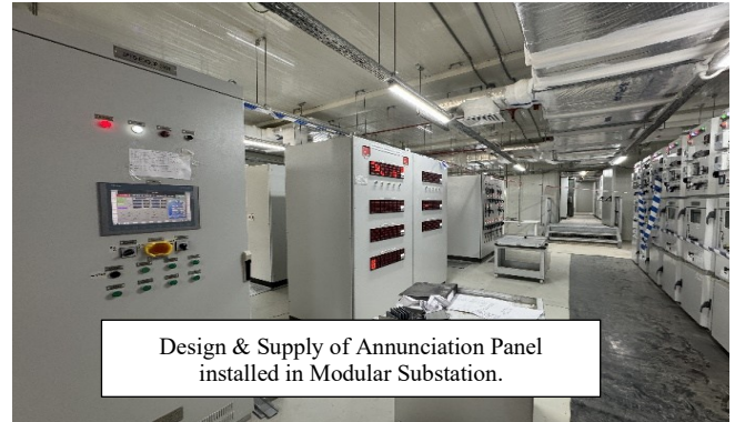
LV Panels and Annunciator Panels
