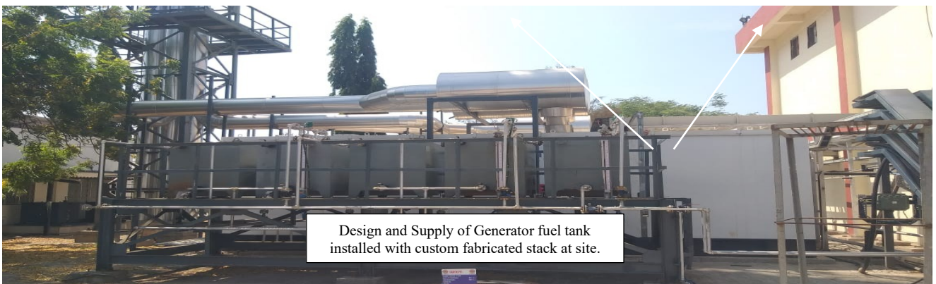
Fuel Tank for Generators
