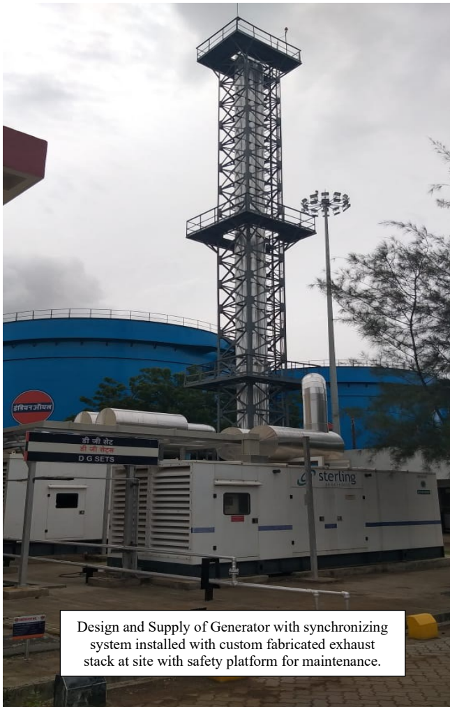
Generator with Exhaust Stack
